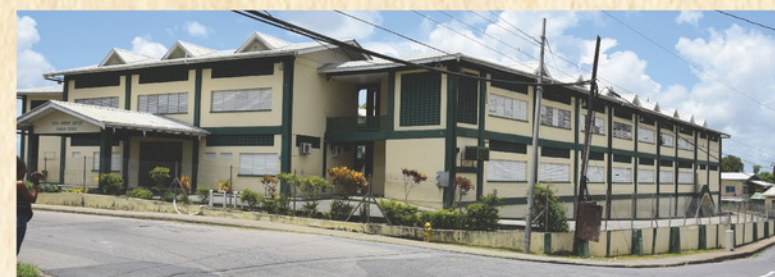
Fifth Company Baptist Primary School
